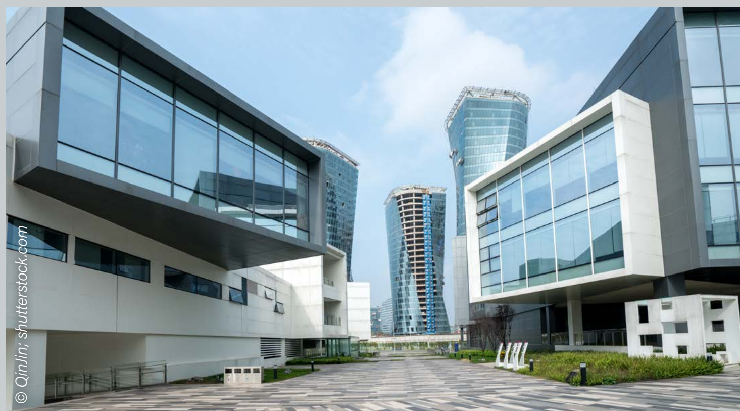
Data centre in Chongqing, China
