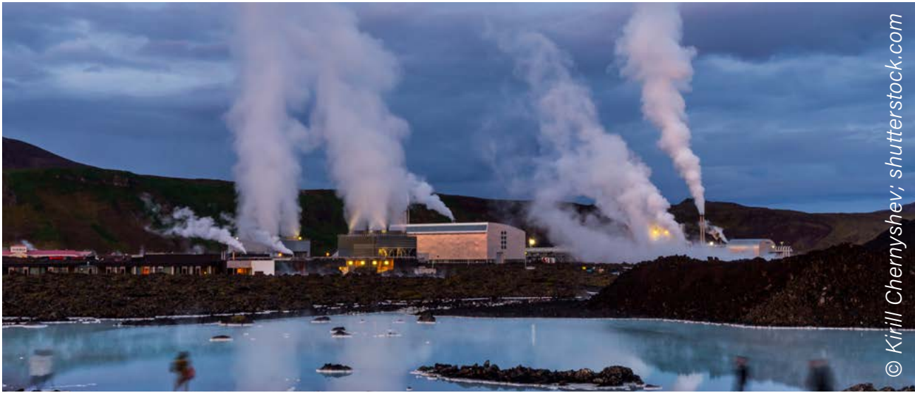
Geothermal Power Plant in Iceland
