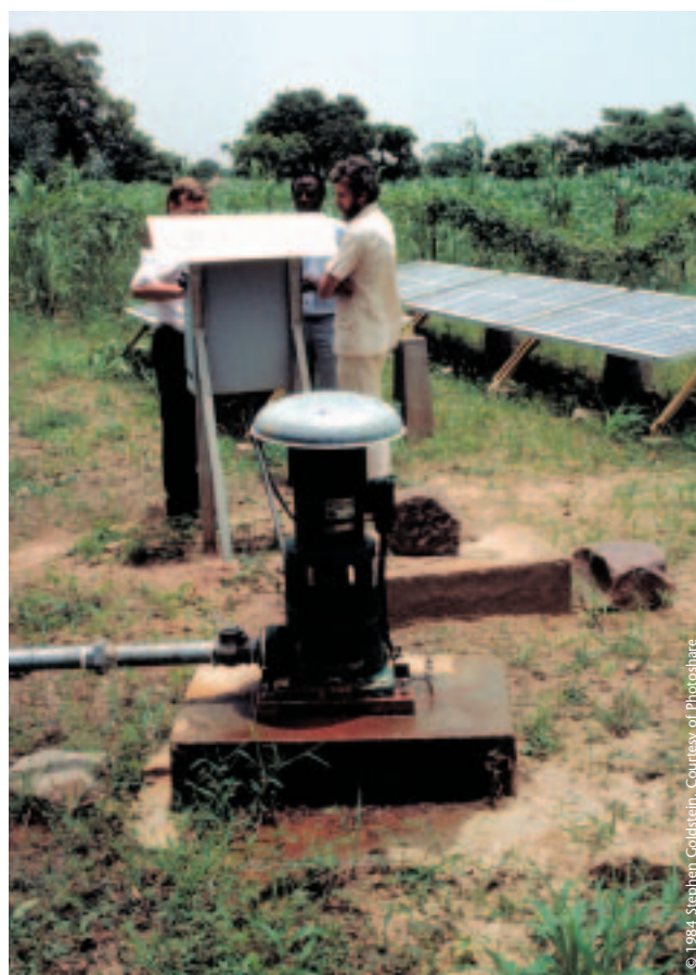
Solar water pumping in Mali
