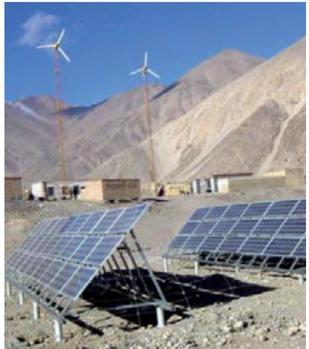
Hybrid mini-grid system powered by wind and solar
