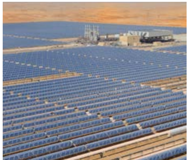
Shams 1 Concentrated Solar Power Plant, Abu Dhabi, UAE
