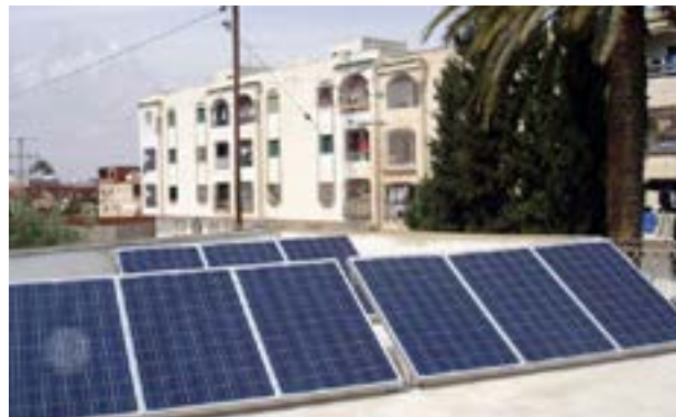
Rooftop PV in Tunisia, Prosol Elec photovoltaic programme for the residential sector
